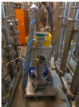
Figure 8: Set-up of the valve test-rig for wet runs in water
