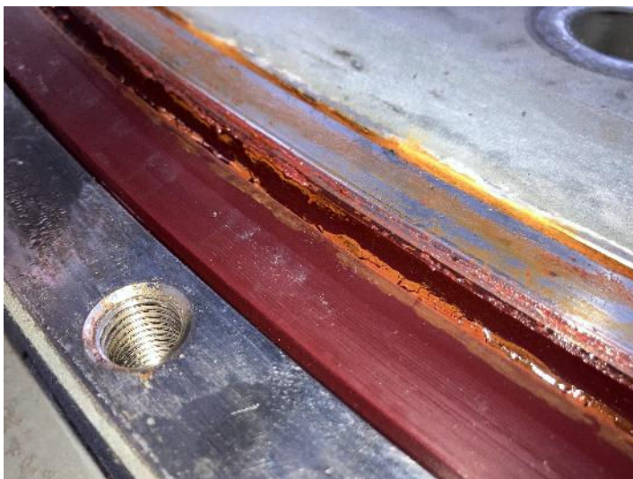
Figure 14: Seal following completion of the test program prior to removal
